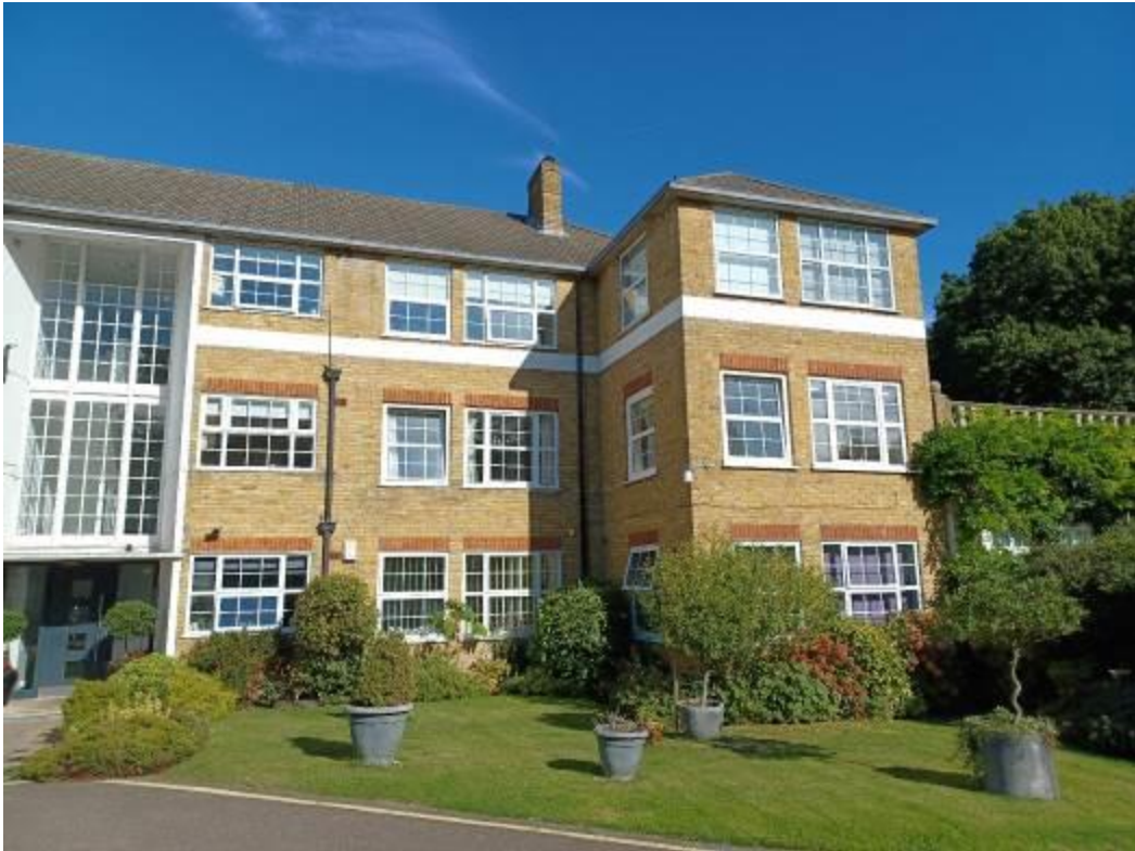
Figure 10. Front elevation of Mulbarton Court, with parapet wall of Barton to the right
